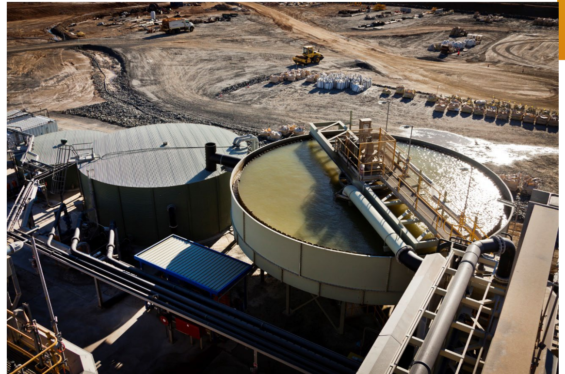
Mineral processing plant at a mine in Western Australia.
